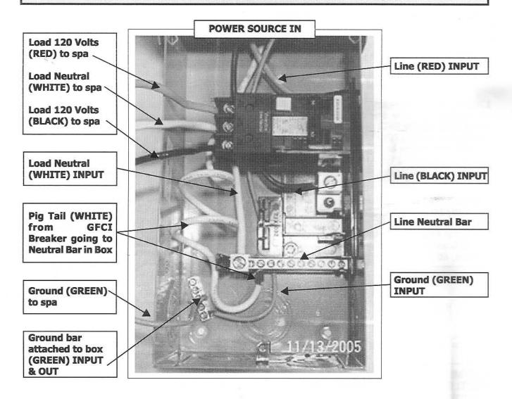
**IMPORTANT NOTE:** Installation of this GFCI — Circuit Breaker, including ampere sizing and selection of conductor size and type — **MUST** be accomplished by a qualified electrician in accordance with the National Electrical Code and all federal, state and local codes and regulations in effect at the time of installation.
